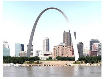
hangs the chain, so stands the arch." In other words, the geometry of a standing arch should mirror that of a hanging chain.
